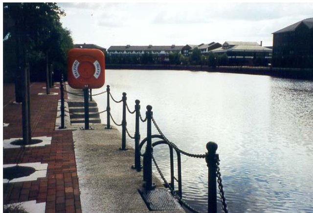
Band 3 solution-Double chain and post with rescue equipment and escape ladders
